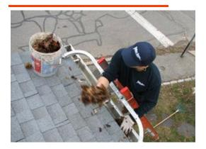
Ice, snow and wind can have devastating consequences. Every winter there is a chance that pipes burst, frozen gutters and other weather-related disasters. Remove leaves, acorns, sticks and other debris from gutters, so melting snow and ice can flow freely. And check your roof insulation. Improper insulation and ventilation in your attic are at the root of most ice daming and gutter back-up causing leaks.
